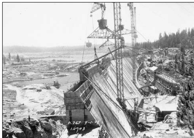
Construction of Shaver Lake Dam at Big Creek, September 1, 1927
