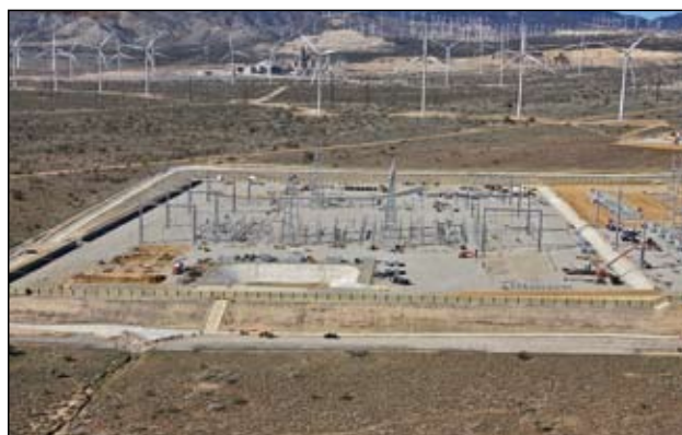
Construction of Windhub Substation, February 10, 2011
